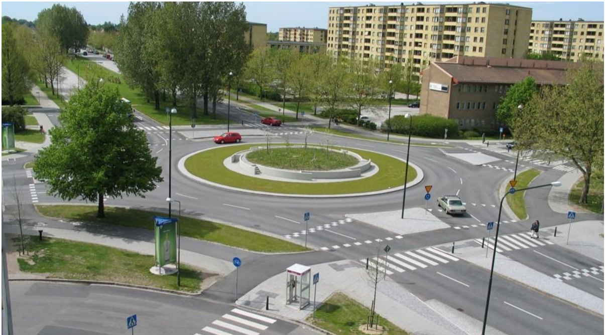
Figure 37 Urban Compact Roundabout
