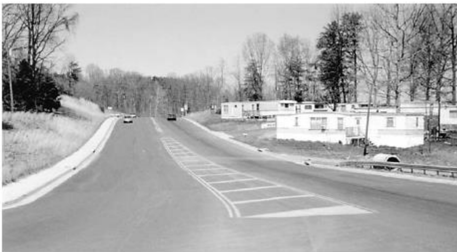
Figure 43 Island Formed by Pavement Markings (Flushed Island)
